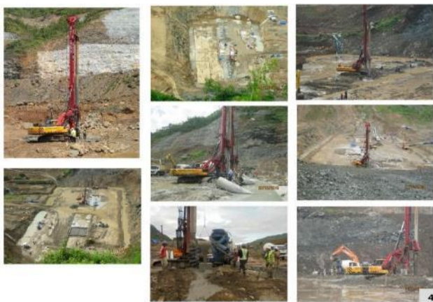
Fig. 6. The Construction of DAM Diaphragm wall
